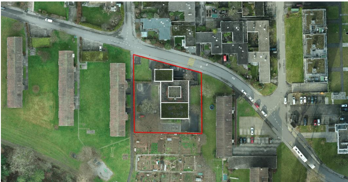
Situation Kindergarten Goldern, General-Guisan-Strasse 26
