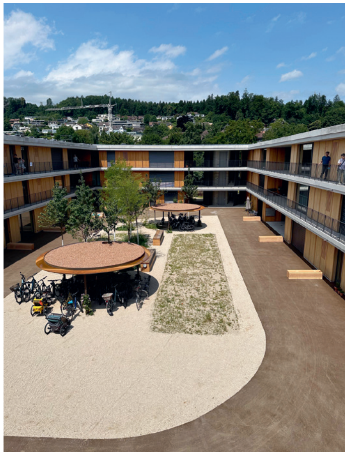
Baufeld 6: Blick in den Innenhof. Foto: Simone Sager-Roth
